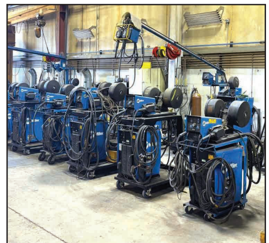
VIEW OF WELDERS
